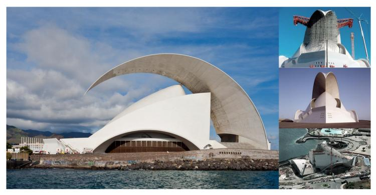
The Tenerife Auditorium is a noteworthy building. The main elements of the building are the auditorium itself and a very large winged element. The structure of the auditorium consists of a circular shell and some shell elements which laterally and partially cover its roof. The large wing starts on the seaward side and rises, supporting itself on the roof of the auditorium and continues as a "flying" cantilever up and over it.
